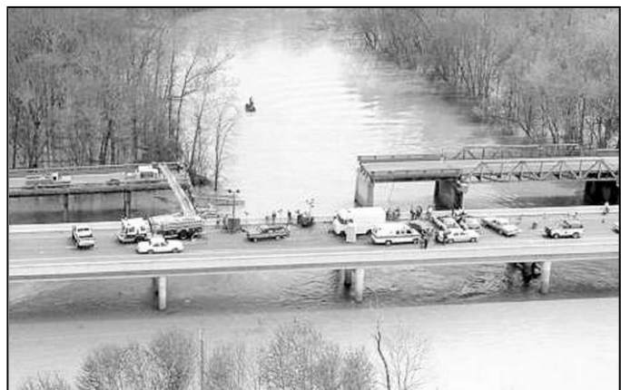
Figure 6-2 US 51 over the Hatchie River
