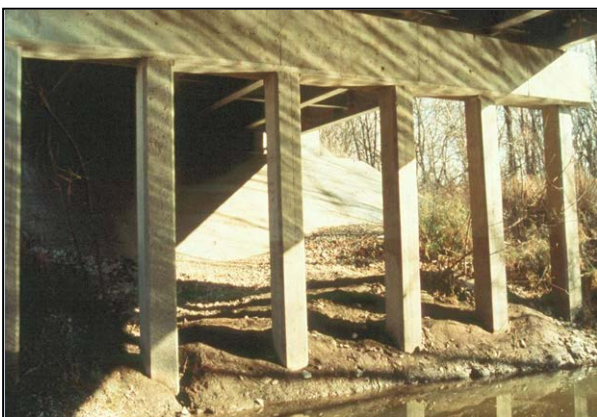
Figure 3-2 Concrete Pile Bent at Low Water
