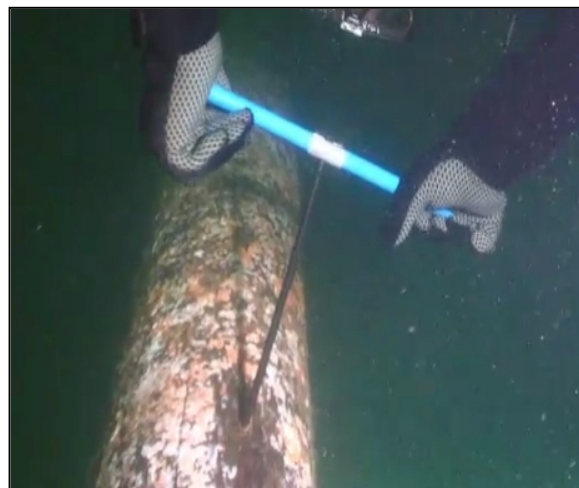
Figure 5-14 Diving Inspector Removing Timber Cores
