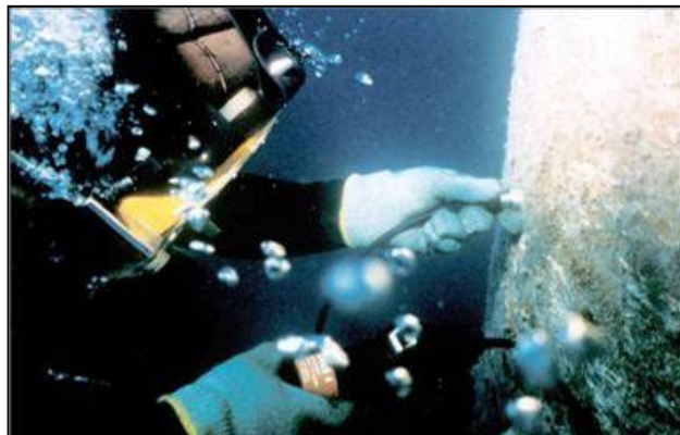
Figure 1-4 Level III Inspection of a Steel Pile with an Ultrasonic Thickness Measuring Device
