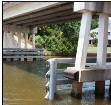
Figure 3-8 Composite Pile and Wale Fender System
