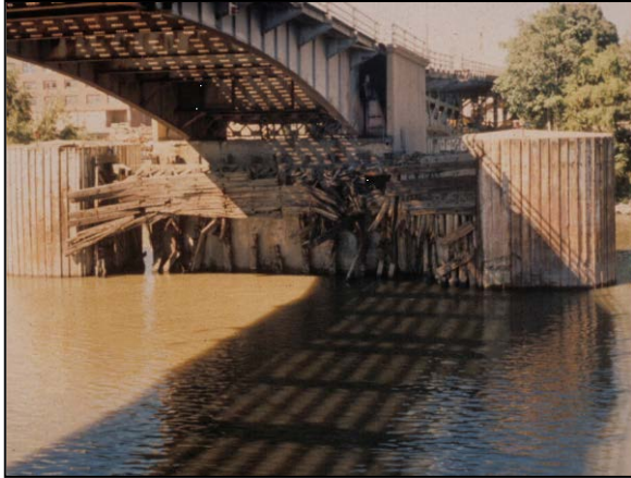
Figure 3-17 Timber Fender System Attached to Pier with Steel Sheet Pile Cell Dolphins
