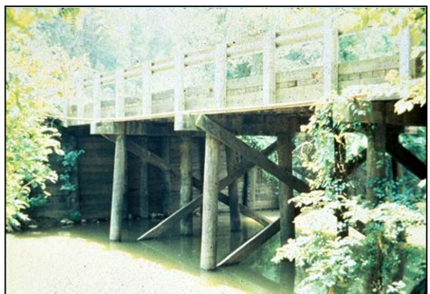
Figure 3-3 Timber Pile Bents and Timber Pile Abutment
