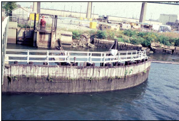
Figure 3-19 Timber Shear Fence
