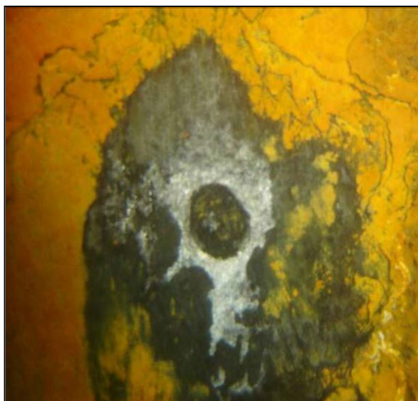
Figure 3-29 Steel Sheet Pile with MIC
