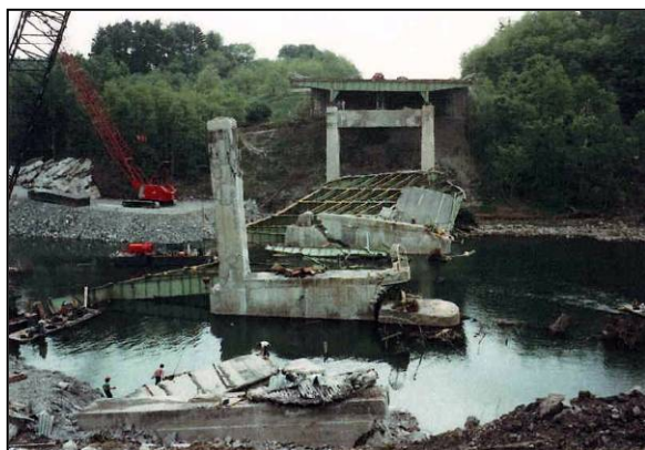
Figure 1-1 I-90 Bridge over Schoharie Creek, New York (1987)
