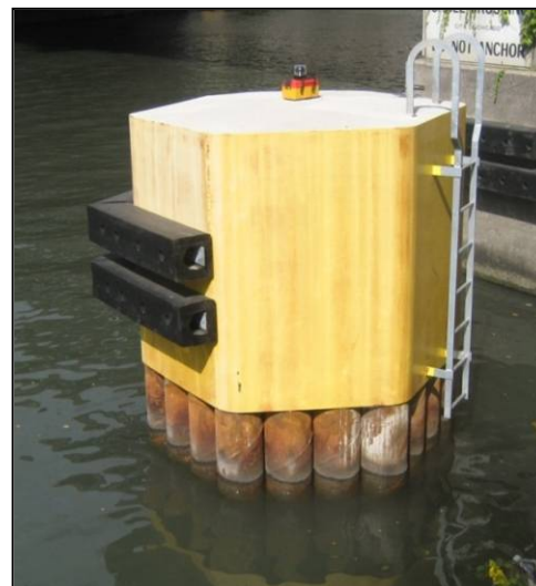
Figure 3-16 Steel Pipe Pile Dolphin with Concrete Cap
