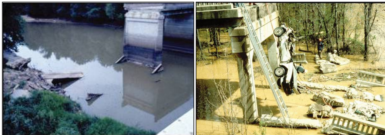
Figure 1-2 US 51 Bridge over Hatchie River, Tennessee (1989)
