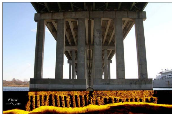
Figure 4-20 Acoustic Image of Concrete Pier with Steel Sheet Piling Cofferdam
