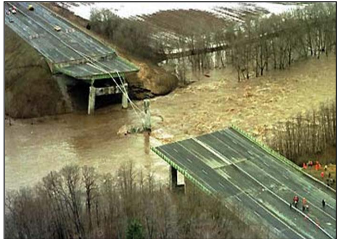
Figure 6-1 I-90 over Schoharie Creek
