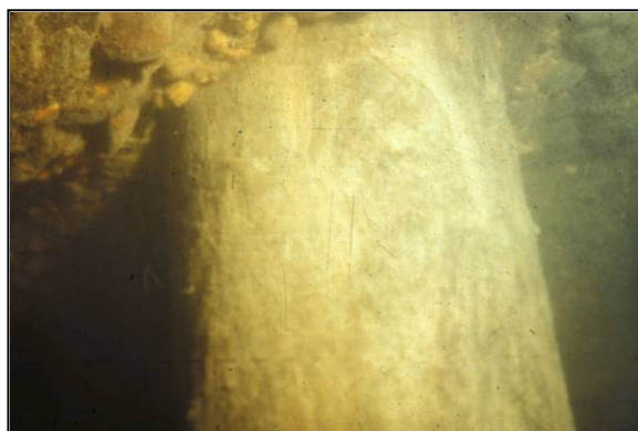
Figure 3-5 Timber Pile at Underside of Concrete Pier
