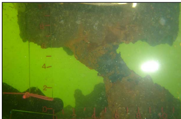
Figure 3-30 Steel Pipe Pile with ALWC
