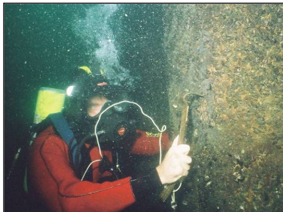
Figure 4-10 Diver Cleaning Submerged Concrete Surface with Hand Scraper
