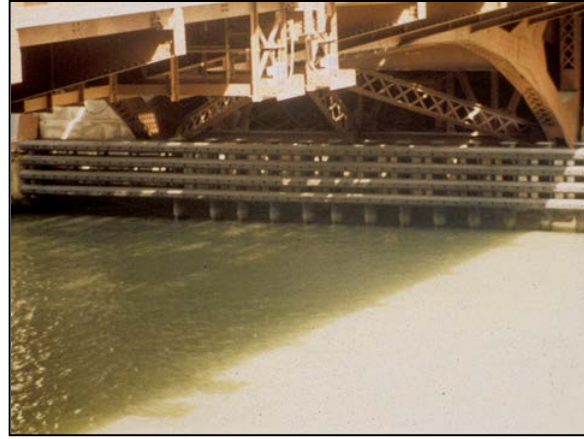
Figure 3-18 Pile Supported Fender System
