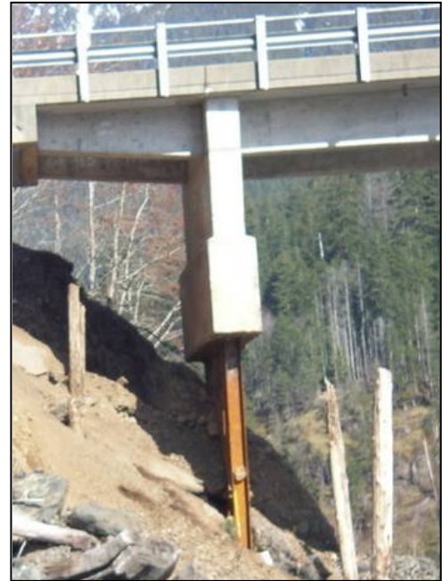
Figure 3-6 Concrete Pier Supported by Steel H-Piles
