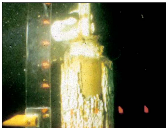
Figure 3-32 Impressed Current Anode
