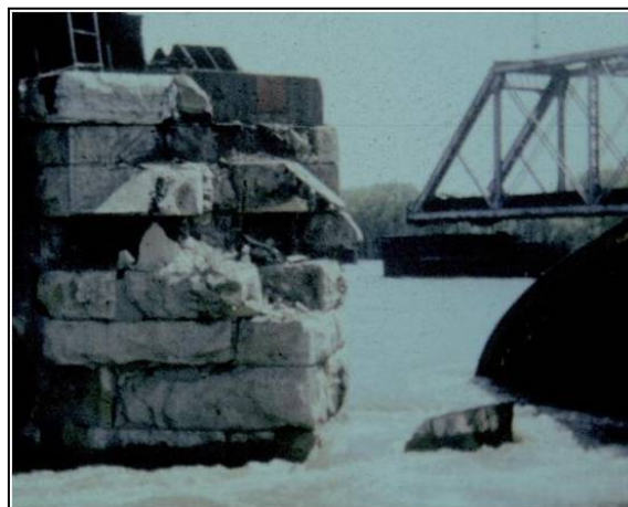
Figure 3-41 Vessel Damage
